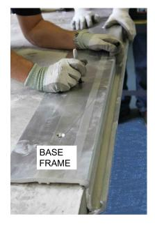
Note: If CS Fire Barrier is to be installed in the joint, please review the Fire Barrier Installation Instructions supplied, and if required install the Fire Barrier BEFORE installation of the Vapor Barrier. The Vapor Barrier should be installed in as long of runs as possible to reduce the number of splices. All sizes of Vapor Barrier are provided in 100' rolls.
