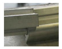
2.3 Place the length of Base Frame along the joint edge installing over the vapor barrier. Fasten the Base Frame with the supplied CS anchors in the predrilled hole locations to the specifications by the anchor manufacture.
