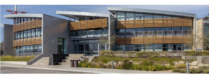
Sun Controls are the best solution for reducing solar heat gain through exterior architectural solar shading. Framed sunshades have a boxier, closed-end aesthetic. Combine blades, screens, and perforated sheet for nearly endless configuration options.
