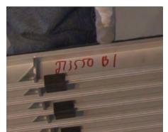
**3** Each grid module is labeled per the drawings to identify location. Begin placing modules in the recess per the shop drawing layout.
