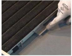
**4** Modules will have spacer clips attached to one side. Spacer clips should face toward adjacent modules.
