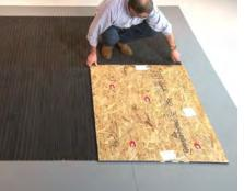
8 If construction is to continue in the building, protect the unit with plywood sheathing.
