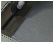
**1** Ensure the recess is flat and smooth. Use non-shrink grout to fill any low spots. Grind down any high spots as well.
