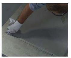
**2** Allow 24 hours for the grout to dry before continuing with the installation.
