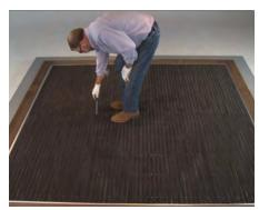
**6** Make final adjustments for rail alignment.
