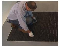
1 Using the supplied shop drawings, place each tagged/numbered module into the recess (or applicable area) as shown on the layout.
