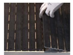
**2** Join modules together by placing the aluminum foot into the black connector.
