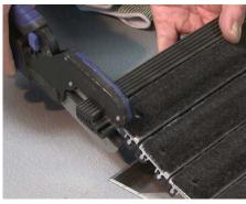
**5** The end trim is shipped oversized to allow for contraction. Cut the end trim flush to the adjacent rail using a utility knife.
