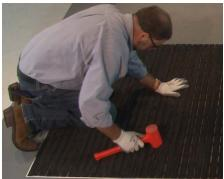
**3** Use a rubber mallet to join the foot into the connector.
