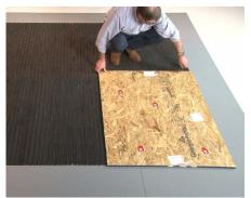
**8** Clean unit with a vacuum. If construction is to continue in the building, protect the unit with plywood sheathing.
