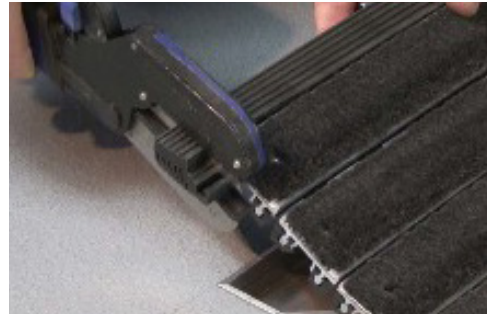
10. Cut the oversized end trim flush to the edge of the rail.
