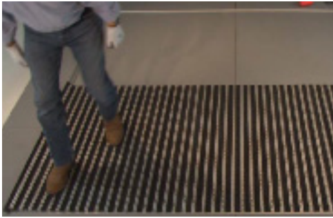
9. Align the mat into the recess.
