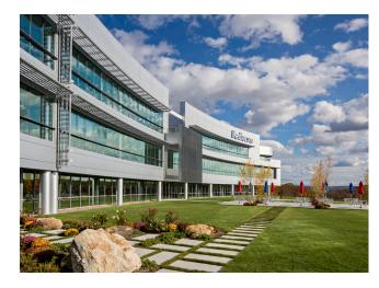
The southwest side of the building features a striking cobalt blue silo, which houses three stories of conference rooms. On the same side the windows are shaded on two levels by Construction Specialties (C/S) 100-3 Cantilevered
