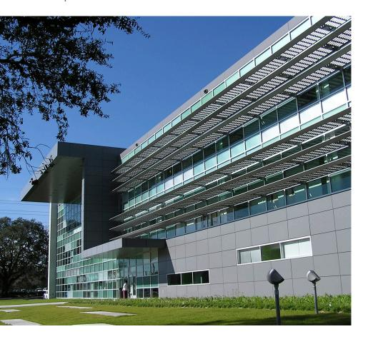
According to Alfonso solar calculations of the 3' deep sunshades proved to be so effective at reducing heat gain that he was able to save the client additional budget dollars by using standard glass instead of the more expensive insulated glass. The C/S Sun Controls reduced the building's energy usage by 18%, and during peak usage 26.4% is saved.
