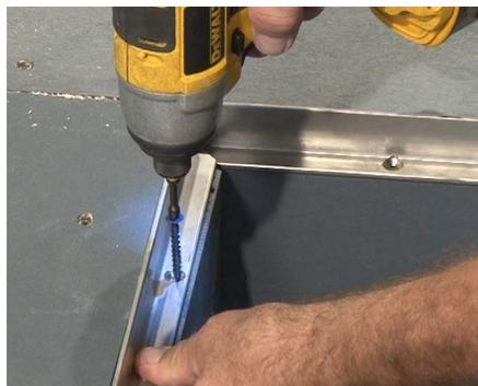
**2** Install the perimeter frame onto the ledge. Use the pre-drilled holes in the frame as a guide and drill into the ledge using a 5/32" drill bit. Fasten the frame using the supplied masonry anchor hardware.
