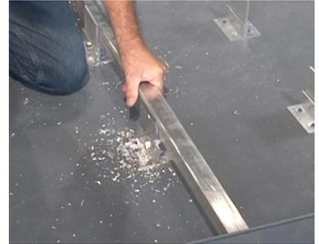
**16** Clamp another continuous support angle to opposite side of the vertical support bar, creating an overall T-shaped support. Drill fastening holes in this angle utilizing the same hole locations previously drilled in the opposing angle.
