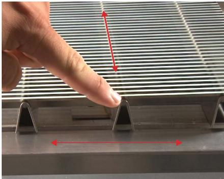
**4** Install the intermediary supports throughout recess. These supports should be installed perpendicular to the support bars attached to the underside of the GridLine material.
