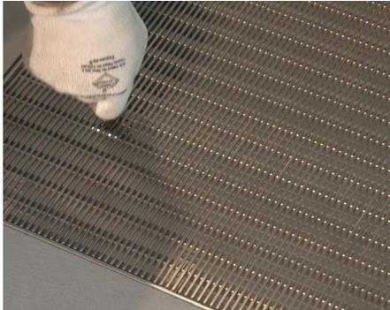
**32** Beginning in the center and working your way out to the edges, **start** the screws with a 1/8" Allen wrench.
