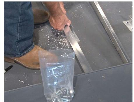
**19** Reinstall the continuous supports in the same T-shape with the vertical support bar located in between. Be sure the angle legs are flush with the top of the vertical support bar and that the drilled holes line up.
