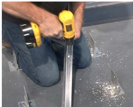
**18** Clamp another continuous support angle to the opposite side of the vertical support bar, creating an overall T-shaped support. Drill fastening holes in this angle utilizing the same hole locations previously drilled in the opposing angle.
