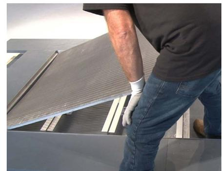
**22** Place the labeled GridLine panels on top of the intermediary supports as shown on the supplied shop drawings.
