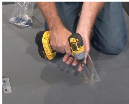
**12** Fasten that new angled leg clip to the floor using the supplied masonry anchors. Repeat at all anchor clip locations.
