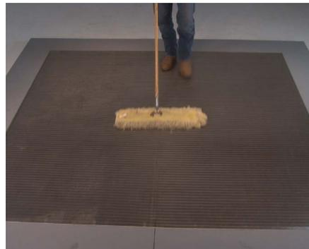
**36** Care & Maintenance: Once the installation is complete, use denatured alcohol to remove the marks on the grids and clean with a mop.
