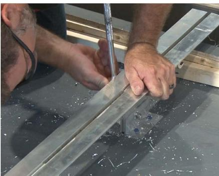
**20** Using a socket/wrench and the supplied nut/bolt hardware, fasten the two continuous support angles to the vertical support bar. Repeat these steps at all angled clip locations.
