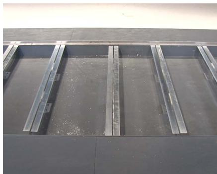
**21** All fully-assembled supports should be installed and flush with the perimeter ledge frame. Now it is time to begin locating the hidden lockdown locations.
