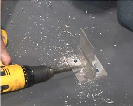
**14** At each clip anchor location use a 5/32" drill bit and drill a hole through both anchor clips and the vertical support bar.
