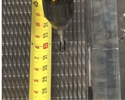
**24** Using a drill or center punch tool, transfer the marked lockdown location to the I-Beam support.
