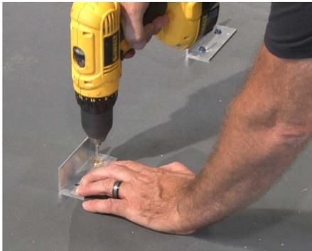
**8** At the module split locations begin by fastening angled clips every 24" along the continuous supports. Use a 5/32" drill bit to make a pilot hole through the pre-drilled holes in the angled leg clips.
