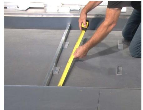
**10** Once intermediary supports are installed at all module splits, measure and install all remaining supports every 18" on center from the module split, in each direction.
