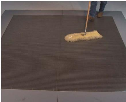
**35** If building construction is to continue, protect the grid with plywood sheathing.
