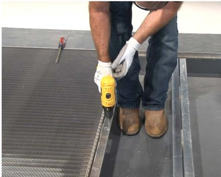
**26** Using a 5/32" drill bit, drill through the support at the locations previously marked from above the panel.
