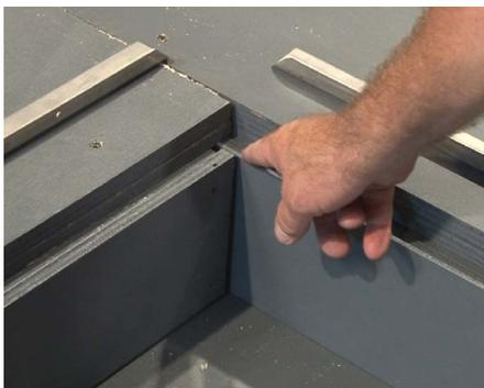
**1** Per the submittal drawings, a ledge should have been created by the concrete installer to install the perimeter frames and form a ledge for the GridLine units to rest upon.
