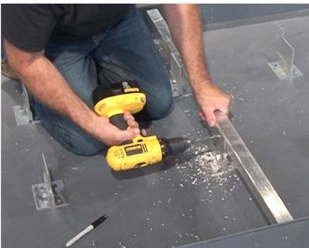
**17** Use a 5/32" drill and drill one pilot hole through the continuous angle and vertical support bar. Repeat this step at all other angled support clip locations.
