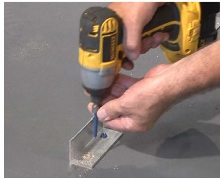
**9** Attach clips to the floor using a driver and the supplied masonry anchor hardware. Repeat at all angled clip locations. Be sure to install all clips facing the same direction.
