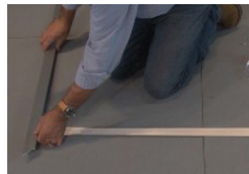
4. Apply the frame to the substrate.
