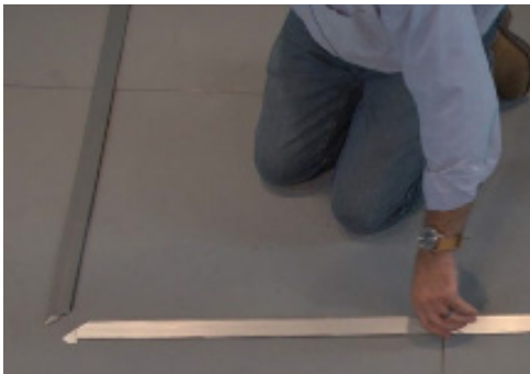
1. Begin by placing the pre-mitered tapered aluminum frame in the correct location.
