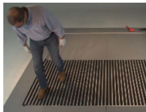
10. Align the mat into the recess.
