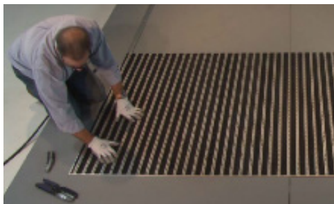
13. For beginners: we recommend using a straight edge to assist in cutting an accurate line. Once the end trim is adjusted, tuck the mat into the recess and push flat.
