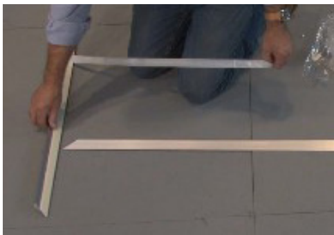
3. Remove backing from the double-sided tape.
