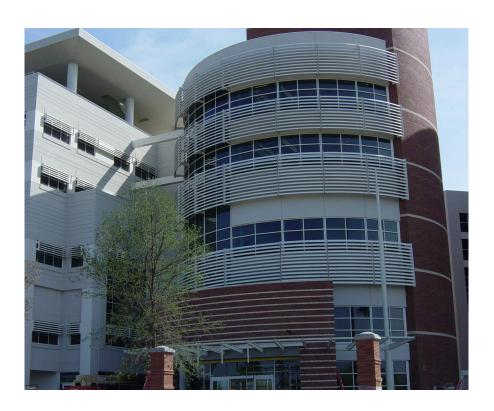
To provide maximum sun control at the entrance to this California Medical Center, RTKL specified a C/S Vertical Sunshade with longspan airfoil blades. The radiused sunshades are anchored to the curtain wall system using tee brackets. On the patient wing C/S Vertical sunshades are used in front of each patient room to reduce heat and glare, while providing natural filtered sunlight into the interior and reducing the need for artificial light.
