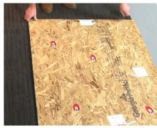
**8** If the building is still under construction, cover the system with plywood sheathing.
