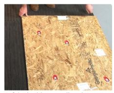
**7** If the building is still under construction, cover the system with plywood sheathing.
