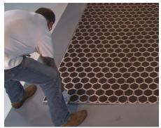
**4** To prepare for adhesive\*, turn the module right side up to access the module's underside. \*Adhesive supplied by others. Recommended brand: 3M #525.
