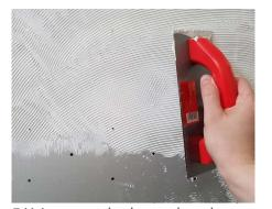
**5** Using a notched trowel apply adhesive evenly across the entire underside of the module. Use an adhesive that is appropriate for bonding aluminum to concrete.
