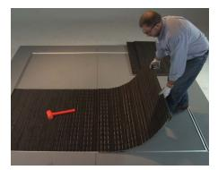
**7** Continue to install the remaining modules into the framed recess.
