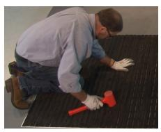
**6** Use a rubber mallet to join the foot into the connector.
