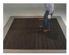
**10** Make final adjustments for rail alignment.
