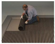
**13** Care & Maintenance: to properly clean underneath the grid and avoid rail damage, roll back the grid edge to the 12th rail. Continue to roll back the grid holding that diameter.
