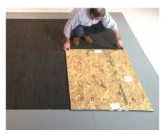
**12** If construction is to continue in the building, protect the unit with plywood sheathing.
