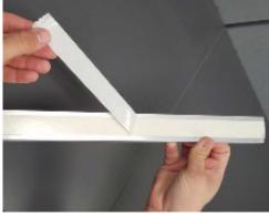
Remove the covering on the tape and reinstall the frame in its correct position and location. Apply pressure on the frame to properly bind the tape to the flooring.
