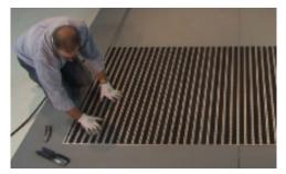
9. For beginners: we recommend using a straight edge to assist in cutting an accurate line. Once the end trim is adjusted, tuck the mat into the recess and push flat.
