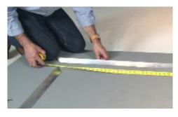
1. Start by dry fitting all frame pieces within the area and use a tape measure to ensure a proper fit. For odd-shaped layouts, match frame tags to the drawing on the pack list.
