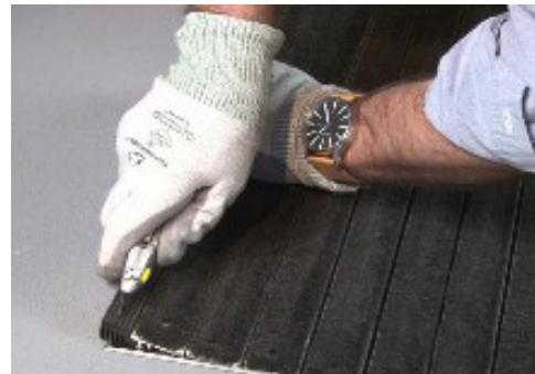
12. For proper overall fit, adjust the end trim using a utility knife with a new, sharp blade. Remove excess trim equally at both ends. The end trim has grooves every 1/8" that you can use to run the blade across.
