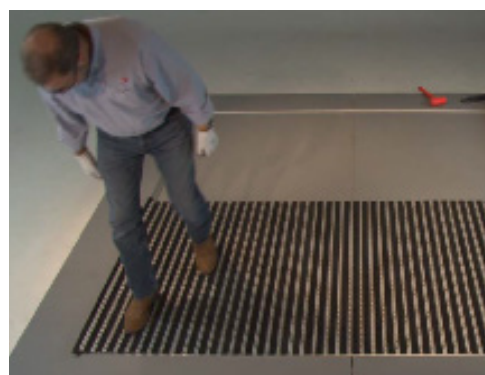
10. Align the mat into the recess.
