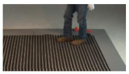
15. Scuff or drag your heel to align the mat. It may be necessary to lift and flap/shake the mat for final alignment.
