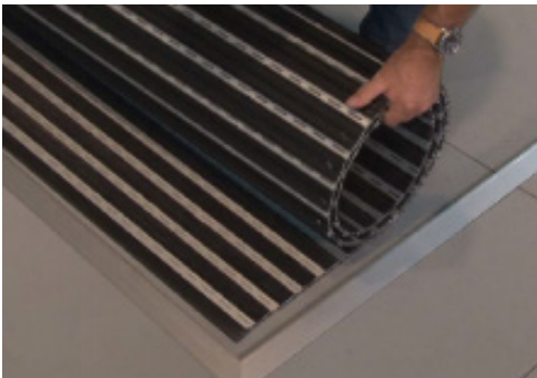
7. After the frame is in place, proceed with the product installation.
