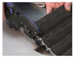
11. Cut the oversized end trim flush to the edge of the rail.
