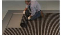
18. Care & Maintenance: to properly clean underneath the mat and avoid rail damage, roll back the mat edge to the 12th rail. Continue to roll back the mat holding that diameter.
