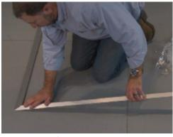
5. Make sure the frame is square and the miters butt properly.
