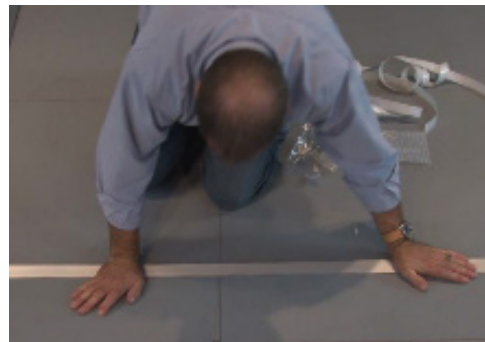
6. Firmly press down on the entire length of the frame to activate the tape.
