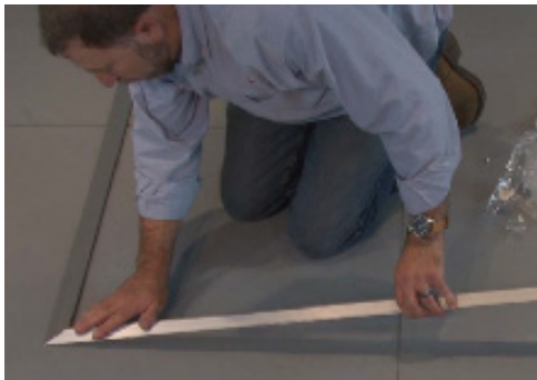
5. Make sure the frame is square and the miters butt properly.
