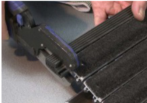
11. Cut the oversized end trim flush to the edge of the rail.
