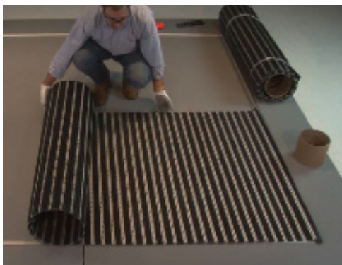
9. Unroll the mats and place into the recess per the drawing layout.
