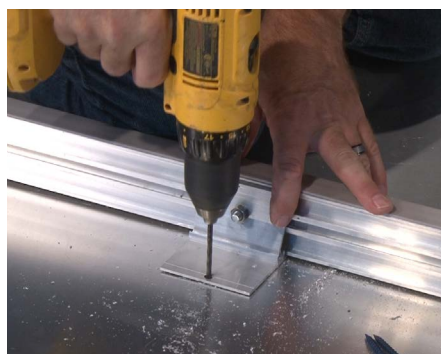
20 Using a 5/16" drill, locate the pre-drilled hole on the horizontal portion of the support clip and drill into the floor.
