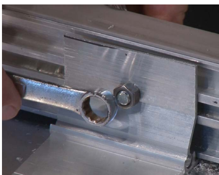
19 Use the supplied bolt, washer and nut hardware with a socket/wrench tool to fasten the vertical portion of the support clip to the support bar.
