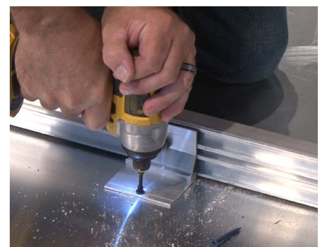
21 Use a driver to install the fastening hardware and secure the support clip to the floor. Clips should be installed alternating on each side of the support.
