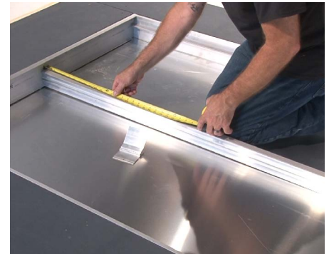
15 To keep intermediary supports from rocking, start at the supports edge and install support clips every 24" along the support, alternating the clip location on each side of the support.
