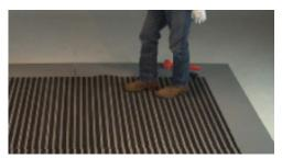
8. Scuff or drag your heel to align the mat. It may be necessary to lift and flap/shake the mat for final alignment.
