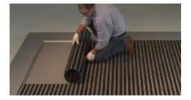
11. Care & Maintenance: to properly clean underneath the mat and avoid rail damage, roll back the mat edge to the 12th rail. Continue to roll back the mat holding that diameter.
