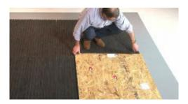
10. If construction is to continue in the building, protect the unit with plywood sheathing.
