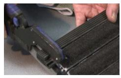
4. Cut the oversized end trim flush to the edge of the rail.
