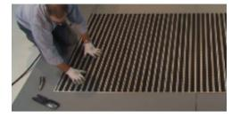
6. For beginners: we recommend using a straight edge to assist in cutting an accurate line. Once the end trim is adjusted, tuck the mat into the recess and push flat.
