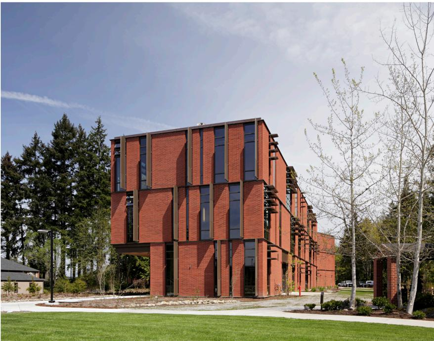
Native mosses cover the roof and C/S Perforated Sun Controls help reduce glare and solar heat gain while still letting diffused daylight enter. Rainwater is collected and diverted into the wetlands. Built with the goal of reducing energy use and dependence on fossil fuels, greenhouse gas emissions and energy consumption, as expected the project is certified LEED Gold.
