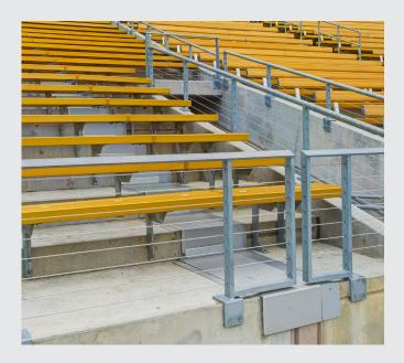
In less than 21 months, we designed, tested, and fabricated custom joint cover assemblies for six seismic joint openings around the stadium that protect the structure and its patrons in the event of an earthquake. Each expansion joint cover had to be custom designed to fit its individual tread and stair riser. The stadium became the first facility to require 12" of expansion, compression, and lateral movement.
