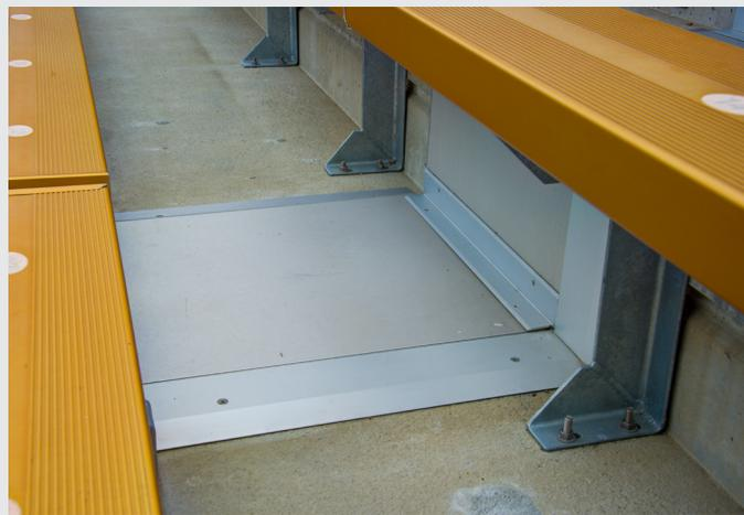
In less than 21 months, we designed, tested, and fabricated custom joint cover assemblies for six seismic joint openings around the stadium that protect the structure and its patrons in the event of an earthquake. Each expansion joint cover had to be custom designed to fit its individual tread and stair riser. The stadium became the first facility to require 12" of expansion, compression, and lateral movement.
