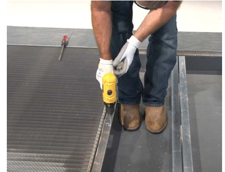
28 Using a 5/32" drill bit, drill through the support at the locations previously marked from above the panel.
