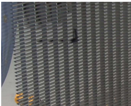
32 Insert a small tool between the marks to later identify the location.
