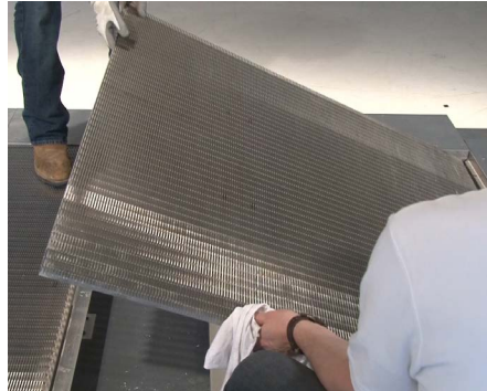
27 Remove the panels to access the supports underneath.
