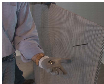
33 On the opposite side, install the hidden lockdown with the small tool acting as the center.
