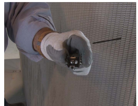
34 Assemble hidden lockdown by inserting the screw through the clip's hole.
