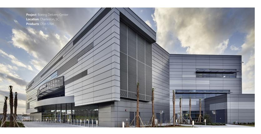
CENTRIA and Construction Specialties have a unique partnership to assure complete integration of CS Louvers and Sun Controls into CENTRIA Formawall Dimension Series Panels and CENTRIA Formavue Windows. CS Louver models include common joinery elements with Formawall Panels to provide a seamless exterior façade.
