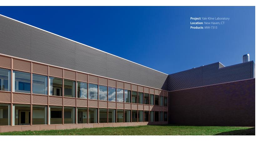
Buildings need to allow fresh air in and keep water out through all weather conditions. The integrated MetalWrap Series Louvers are designed for use in large areas where both louver performance and insulated walls are required. These systems utilize Storm Resistant Louvers in active louver areas and CENTRIA MetalWrap Series insulated back up panel systems at inactive areas.
