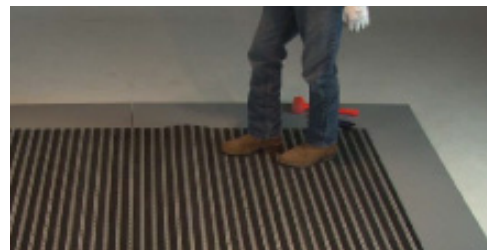
14. Scuff or drag your heel to align the mat. It may be necessary to lift and flap/shake the mat for final alignment.
