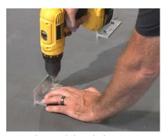
11 At the module split locations begin by fastening angled clips every 24" along the continuous supports. Use a 5/32" drill bit to make a pilot hole through the pre-dilled holes in the angled leg clips.
