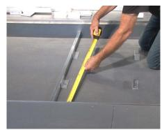
**13** Once intermediary supports are installed at all module splits, measure and install all remaining supports every 18" on center from the module split, in each direction.
