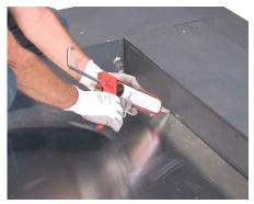
**6** Use silicone caulking to caulk the recess' perimeter seams and any seam where multiple pan sheets abut.
