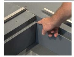
1 Per the submittal drawings, a ledge should have been created by the concrete installer to install the perimeter frames and form a ledge for the GridLine units to rest upon.
