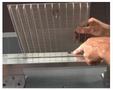
**30** Place the grid module with the installed clip/tab hardware into its corresponding Tinnerman clip location.
