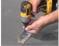
**12** Attach clips to the floor using a driver and the supplied masonry anchor hardware. Repeat at all angled clip locations. Be sure to install all clips facing the same direction.
