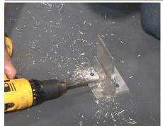
**17** At each clip anchor location use a 5/32" drill bit and drill a hole through both anchor clips and the vertical support bar.
