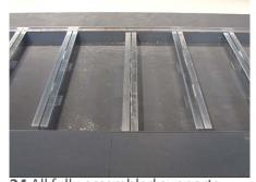
**24** All fully-assembled supports should be installed and flush with the perimeter ledge frame. Now it is time to begin locating the hidden lockdown clips.
