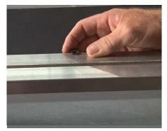
**28** Install one Tinnerman clip at each drilled location along the supports.
