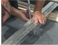
23 Using a socket/wrench and the supplied nut/bolt hardware, fasten the two continuous support angles to the vertical support bar. Repeat these steps at all angled clip locations.
