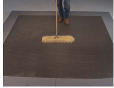
**36** Care & Maintenance: Once the installation is complete, use denatured alcohol to remove the marks on the grids and clean with a mop.
