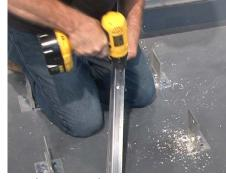
21 Clamp another continuous support angle to the opposite side of the vertical support bar, creating an overall T-shaped support. Drill fastening holes in this angle utilizing the same hole locations previously drilled in the opposing angle.
