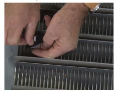
**29** Mount the screw into the welded tab. Use electrical tape to hold the screw in place.
