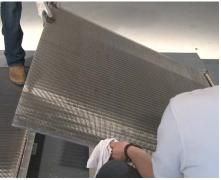
**25** Remove the panels to access the supports underneath.
