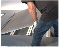
**25** Place the labeled GridLine panels on top of the intermediary supports as shown on the supplied shop drawings.
