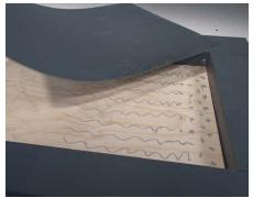
**5** Place the pre-sized drain pan sheet(s) into the recess. Apply pressure evenly over the drain pan material to properly bond into the recess.
