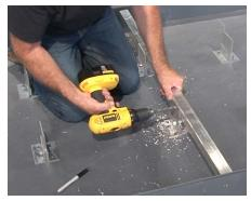
**20** Use a 5/32" drill and drill one pilot hole through the continuous angle and vertical support bar. Repeat this step at all other angled support clip locations.
