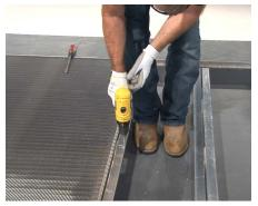
**26** Using a 5/32" drill bit, drill through the support at the locations previously marked from above the panel.
