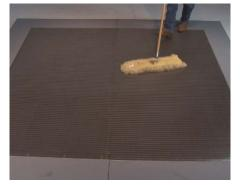
**35** If building construction is to continue, protect the grid with plywood sheathing.
