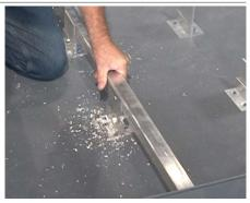
19 Clamp one continuous support angle onto a vertical support bar. The angle should be positioned so one leg is tight against, and parallel with the vertical support bar. The other leg should be facing away from the vertical support bar. The top of this leg should be flush with the perimeter ledge frame.
