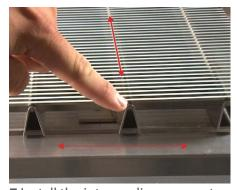
7 Install the intermediary supports throughout recess. These supports should be installed perpendicular to the support bars attached to the underside of the GridLine material.
