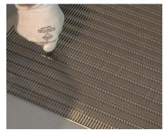
**32** Beginning in the center and working your way out to the edges, **start** the screws with a 1/8" Allen wrench.
