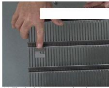
23 The lockdowns are already located and pre-installed on the grid module. Lockdowns are not required along the perimeter ledge frame.
