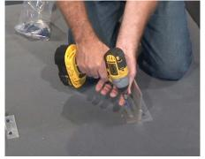
**15** Fasten that new angled leg clip to the floor using the supplied masonry anchors. Repeat at all anchor clip locations.
