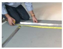
1. Start by dry fitting all frame pieces within the area and use a tape measure to ensure a proper fit. For odd-shaped layouts, match frame tags to the drawing on the pack list.
