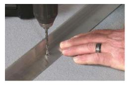
3. Using the 5/2" masonry bit, drill into the concrete 24" on center. Fasten the frame with the supplied masonry anchors using a #2 Phillips-head screwdriver.
