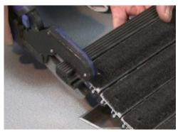
7. Cut the oversized end trim flush to the edge of the rail.
