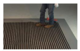
11. Scuff or drag your heel to align the mat. It may be necessary to lift and flap/shake the mat for final alignment.
