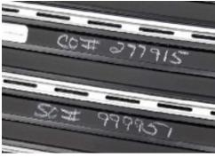
4. For layout sequence of the mat units with multiple sections, refer to the shop drawings and the mark numbers placed on the backside of the mats.
