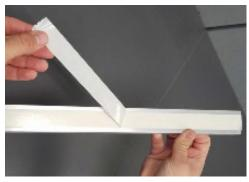
3. Remove the covering on the tape and reinstall the frame in its correct position and location. Apply pressure on the frame to properly bind the tape to the flooring.
