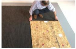
13. If construction is to continue in the building, protect the unit with plywood sheathing.
