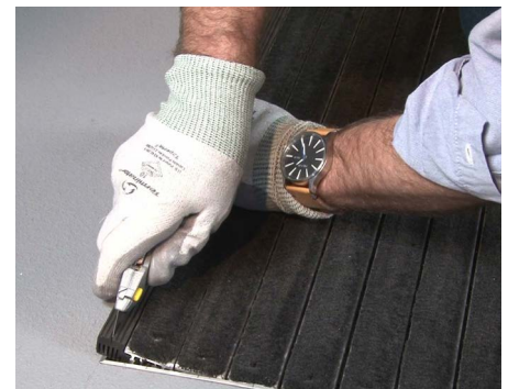
12 For proper fit, the end trim can be cut in any of the grooves that are spaced 1/8" apart using a sharp utility knife. Score several times to cut
