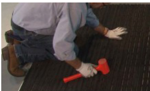
9. Use a rubber mallet to join the foot into the connector.
