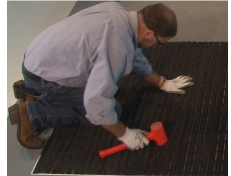
9 Use a rubber mallet to join the foot into the connector.
