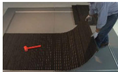
10. Continue to install the remaining modules.
