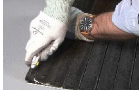
12. For proper fit, the end trim can be cut in any of the grooves that are spaced 1/8" apart using a sharp utility knife. Score several times to cut.
