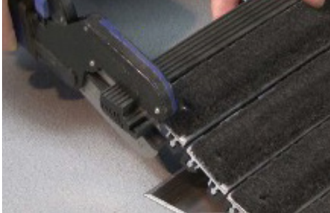
11. The end trim is shipped oversized to allow for contraction. Cut the end trim flush to the adjacent rail using a utility knife.
