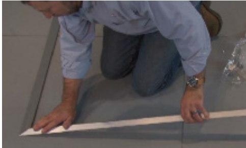
5. Make sure the frame is square and the miters butt properly.
