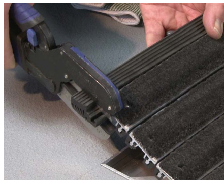
11 The end trim is shipped oversized to allow for contraction. Cut the end trim flush to the adjacent rail using a utility knife.
