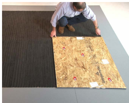
14 Clean the unit with a vacuum. If construction is to continue in the building, protect the unit with plywood sheathing.
