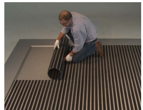
15 Care & Maintenance: to properly clean underneath the grid and avoid rail damage, roll back the grid edge to the 12th rail. Continue to roll back the grid holding that diameter.
