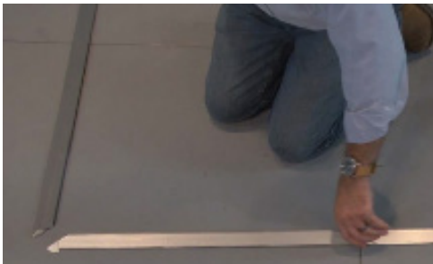
1. Place the pre-mitered tapered aluminum frame at the correct floor location.
