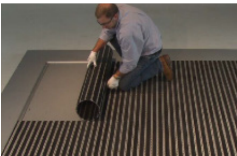
15 Care & Maintenance: to properly clean underneath the grid and avoid rail damage, roll back the grid edge to the 12th rail. Continue to roll back the grid holding that diameter.
