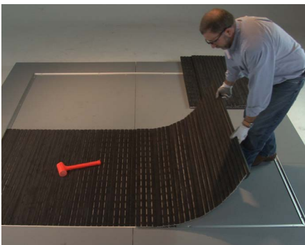
10 Continue to install the remaining modules.
