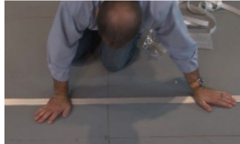
6. Firmly press down on the entire length of the frame to activate the tape.
