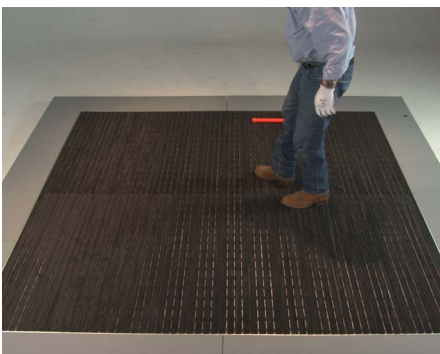
13 Make final adjustments for rail alignment.
