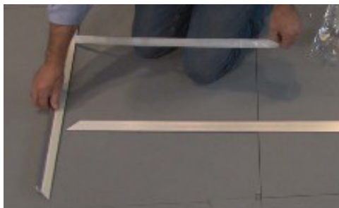
3. Remove the backing from the double-sided tape.
