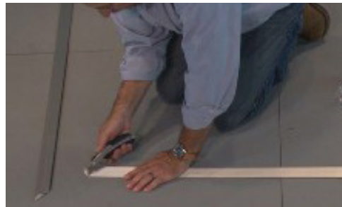
2. Prepare the flooring surface to allow the tape to properly bond to the floor.
