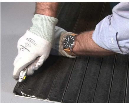
**10** For proper fit, the end trim can be cut in any of the grooves that are spaced 1/8" apart using a sharp utility knife. Score several times to cut completely through the material.
