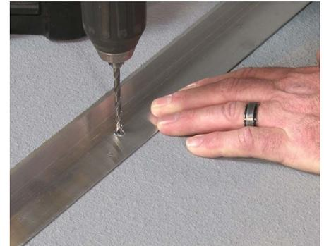
**3** Using the 5/32" masonry bit, drill into the concrete 24" on center. Fasten the frame with the supplied masonry anchors using a #2 Phillips-head screwdriver.
