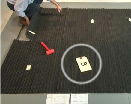
**4** Grid modules are tagged alphabetically in order of placement. Install into the recess accordingly. For odd-shaped layouts, refer to the supplied shop drawings.
