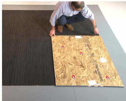
**20** Clean the unite with a vacuum. If construction is to continue in the building, protect the unit with plywood sheathing.
