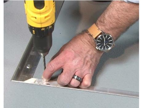
**15** Using 5/32" masonry drill bit, drill out both holes for the locator bar anchors to center the supplied locator bars on the lines marked on the floor.
