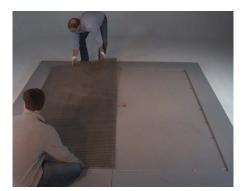
**12** Dry fit all grid modules into the area per the supplied shop drawings.
