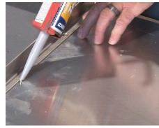
**11** Use silicone caulking to caulk the recess' perimeter seams and any seam where multiple pan sheets abut.
