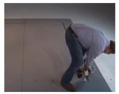
**4** Use a 5/32" masonry bit to drill into the substrate at each welded tab hole for the anchor.
