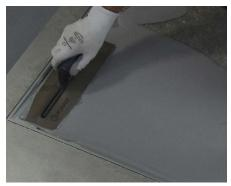
**6** To make the sub-floor level with the bottom frame leg, use non-shrink grout and trowel flush with the top of the bottom leg of the level base frame.
