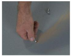
**19** Insert the lead shield with the cone portion going into the hole first.
