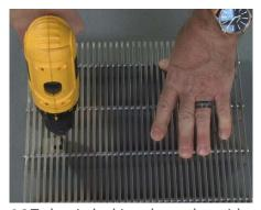
**16** To begin locking down the grid, make sure the grid modules are aligned and transfer the mark for the anchor to the substrate using a 1/8" drill bit. Repeat for each lockdown.
