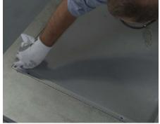
**8** Use a rag to clean the excess grouting from the top of the frame leg. Allow 24 hours for the grout to dry before continuing with the installation.
