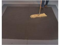
25 Care & Maintenance: Once the installation is complete, use denatured alcohol and a mop to clean the grid surface. If building construction is to continue, protect the grid with plywood sheathing.
