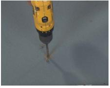
**17** With a masonry bit, drill a 3/8" hole, 5/8" deep.
