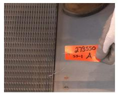
**13** Each module is tagged identify a specific location per the drawing.
