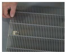
**22** Flip the grid over and align all screws into the lead shields.
