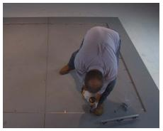
**5** Screw the supplied masonry anchors into the pre-drilled holes to attach the frame.
