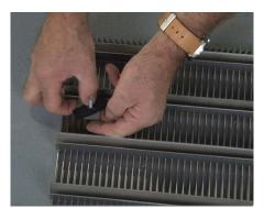
**21** Mount the screw into the welded tab. Use electrical tape to hold the screw in place. Repeat for each lockdown.
