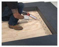
**9** Proceed to the drain pan installation. Use a caulk gun to apply adhesive on top of the newly grouted area.
