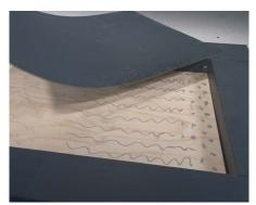
**10** Place the pre-sized drain pan sheet(s) into the recess. Apply pressure evenly over the drain pan material to properly bond into the recess inside of the perimeter frame legs.
