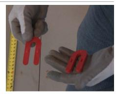
**3** It may be necessary to use shims to set the frame flush with the finished floor.
