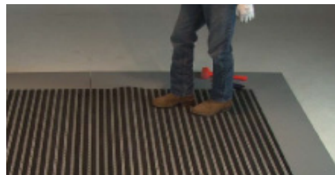
8. Scuff or drag your heel to align the mat. It may be necessary to lift and flap/shake the mat for final alignment.
