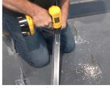
21 Clamp another continuous support angle to the opposite side of the vertical support bar, creating an overall T-shaped support. Drill fastening holes in this angle utilizing the same hole locations previously drilled in the opposing angle.
