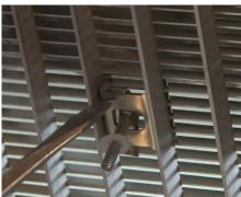
**40** Use a screwdriver to seat the hook of the clip around the support bar.
