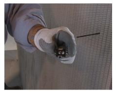
**37** Assemble hidden lockdown by inserting the screw through the clip's hole.
