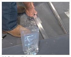
22 Reinstall the continuous supports in the same T-shape with the vertical support bar located in between. Be sure the angle legs are flush with the top of the vertical support bar and that the drilled holes line up.
