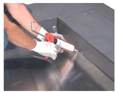
**6** Use silicone caulking to caulk the recess' perimeter seams and any seam where multiple pan sheets abut.
