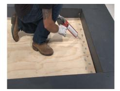
**4** Begin the installation by installing the drain pans into the recess. Use a caulk gun to apply adhesive on top of the concrete surface throughout the entire recess.
