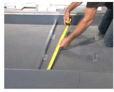
**13** Once intermediary supports are installed at all module splits, measure and install all remaining supports every 24" on center from the module split, in each direction.
