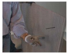
**36** On the opposite side, install the hidden lockdown with the small tool acting as the center.
