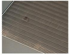
**46** Go back to the center and **lightly draw down** the screws, working your way out to the edges.
