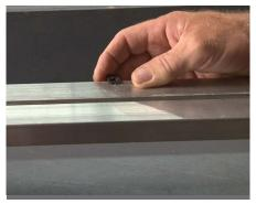
**33** Install one Tinnerman clip at each drilled location along the supports.
