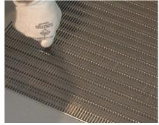
**45** Beginning in the center and working your way out to the edges, **start** the screws with a 1/8" Allen wrench.
