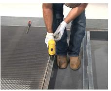
**31** Using a 5/32" drill bit, drill through the support at the locations previously marked from above the panel.
