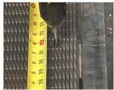
**29** Using a drill or center punch tool, transfer the marked lockdown location to the I-Beam support.
