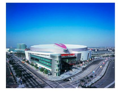
The Staples Center features a sloping roof and tilted walls. Over 400 sq. ft. of louvers were custom manufactured to the exact dimensions to align properly with the tilted wall condition. 11' tall trapezoidal louvers can be found on all sides of the center. At the office and retail entrance, an elliptical tower houses a C/S Vert-A-Cade 300 roof screen to provide ventilation to the HVAC equipment. C/S louver blades were stretch-formed to provide proper blade alignment on all sides of the ellipse.
