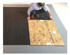
**24** If building construction is to continue, protect the grid with plywood sheathing.
