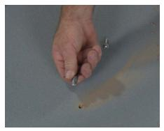
**15** Insert the lead shield with the cone portion going into the hole first.
