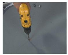
**13** Remove the grid panel and begin drilling the lockdown holes using a masonry bit. Drill a 3/8" hole, 5/8" deep.
