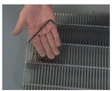
**20** Beginning in the center of the grid module and working your way out to the edges, **start** the screws using an 1/8" Allen wrench.
