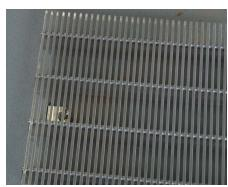
**19** To finish the grid panel installation, flip the grid over and align all screws into the lead shields.
