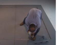
**5** Fasten the supplied masonry anchors into the pre-drilled holes to attach the frame.
