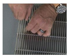
**21** Go back to the center and **lightly draw down** the screws, working your way out to the edges.
