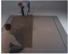
**8** Dry fit all grid modules into the area per the supplied shop drawings.
