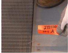
**9** Each module is tagged identify a specific location per drawing.
