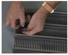
17 Insert the mounting (or fastening screw) into the welded tab lockdown. Use a piece of electrical tape to hold the screw in place.
