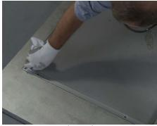
**7** Use a rag to clean the excess grouting from the top of the frame leg. Allow 24 hours for the grout to dry before continuing with the installation.
