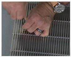
**22** Go back to the center and **tighten** the screws, working your way out to the edge. Repeat this process for the remaining modules.
