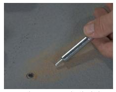
**16** Use the setting tool to lock the shield.
