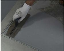
6 To make the sub-floor level with the bottom frame leg, use non-shrink grout (Quikrete 1585 or similar) and trowel flush with the top of the bottom leg of the level base frame. The recess should be smooth and flat.
