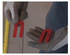
**3** It may be necessary to use shims to set the frame flush with the finished floor.
