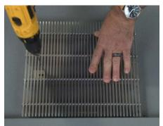
**12** To begin locking down the grid, make sure the grid modules are aligned and transfer the mark for the anchor to the substrate using a 1/8" drill bit or a center punch tool. Repeat for each lockdown location.
