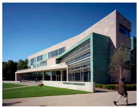
The architect specified 10" C/S Horizontal Airfoil blades to be mounted directly to the vertical curtainwall mullions via cut aluminum brackets. The narrow blade spacing is designed to limit direct sun from entering the student center's South facing window wall. The sunshades reduce the heat and glare getting into the building and lessen the load on the HVAC.
