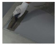
**4** To make the subfloor level with the bottom frame leg, use nonshrink grout and trowel flush with the top of the bottom leg of the level base frame.
