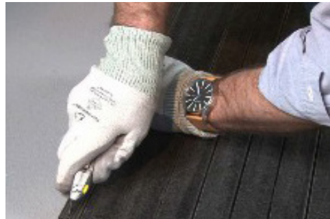
12. For proper fit, the end trim can be cut in any of the grooves that are spaced 1/8" apart using a sharp utility knife. Score several times to cut.
