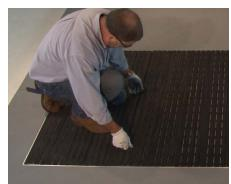
**7** Place modules in proper place as shown on the shop drawings.
