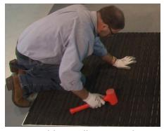
**9** Use a rubber mallet to join the foot into the connector.
