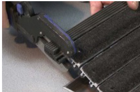
11. The end trim is shipped oversized to allow for contraction. Cut the end trim flush to the adjacent rail using a utility knife.
