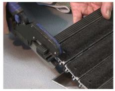
11 The end trim is shipped oversized to allow for contraction. Cut the end trim flush to the adjacent rail using a utility knife.
