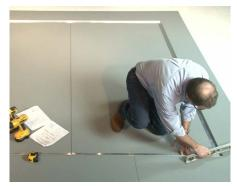
**2** Using a straight edge, ensure the top frame edge is flush with the surrounding floor surface. Shim frame every 24" if necessary to achieve required height.
