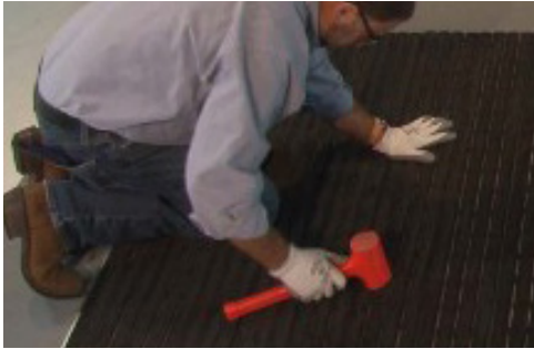
9. Use a rubber mallet to join the foot into the connector.
