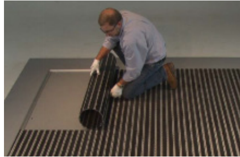
16. Care & Maintenance: to properly clean underneath the grid and avoid rail damage, roll back the grid edge to the 12th rail. Continue to roll back the grid holding that diameter.
