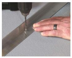
**3** Using the 5/32" masonry bit, drill into the concrete 24" on center. Fasten the frame with the supplied masonry anchors using a #2 Phillips-head screwdriver.
