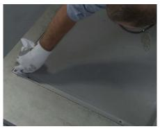
**6** Use a rag to clean the excess grouting from the top of the frame leg. **Allow 24 hours for the grout to dry** before cotinuing with the installation.
