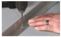
3. Using the ⅓₂″ masonry bit, drill into the concrete 24" on center. Fasten the frame with the supplied masonry anchors using a #2 Phillips-head screwdriver.
