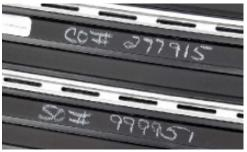
4. For layout sequence of the mat units with multiple sections, refer to the shop drawings and the mark numbers placed on the backside of the mats.
