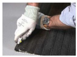
8. For proper overall fit, adjust the end trim using a utility knife with a new, sharp blade. Remove excess trim equally at both ends. The end trim has grooves every 1/8" that you can use to run the blade across.
