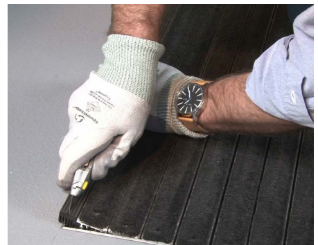
9 For proper fit, the end trim can be cut in any of the grooves that are spaced 1/8" apart using a sharp utility knife. Score several times to cut
