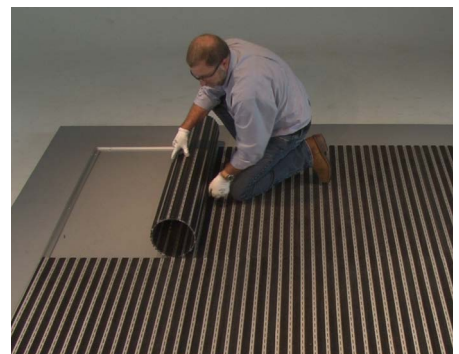
12 Care & Maintenance: to properly clean underneath the grid and avoid rail damage, roll back the grid edge to the 12th rail. Continue to roll back the grid holding that diameter.
