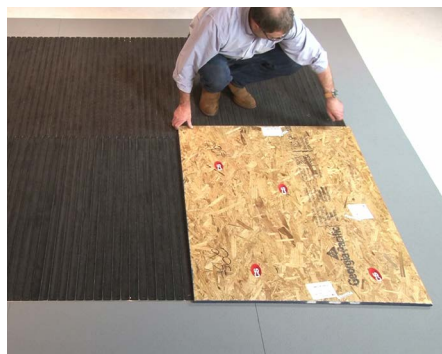
11 Clean unit with a vacuum. If construction is to continue in the building, protect the unit with plywood sheathing.
