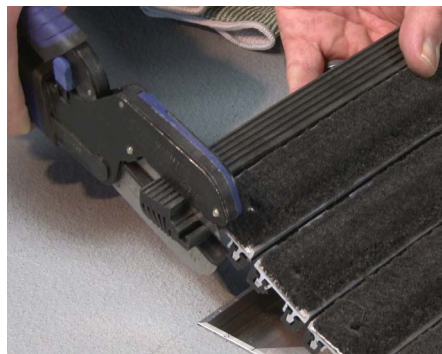
8 The end trim is shipped oversized to allow for contraction. Cut the end trim flush to the adjacent rail using a utility knife.
