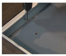
**5** Using a 5/16" masonry bit, drill into the concrete every 24" center. Fasten the frame with the supplied masonry anchors using a #2 Phillips-head screwdriver.
