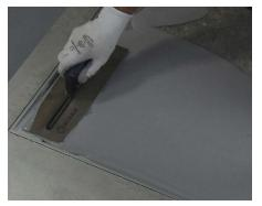
**7** To make the sub-floor level with the bottom frame leg, use non-shrink grout and trowel flush with the top of the bottom leg of the level base frame.
