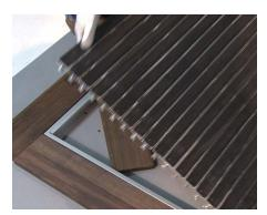
**16** Care & Maintenance: to clean beneath the grid, use a slotted screwdriver to remove grid. Place wood blocking under grid and remove panels.
