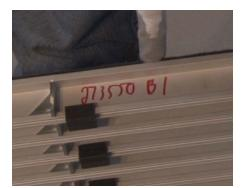
**10** Each grid module is labeled per the drawings to identify location. Begin placing modules in the recess per the shop drawing layout.
