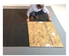
**15** If construction is to continue in the building, protect the unit with plywood sheathing.
