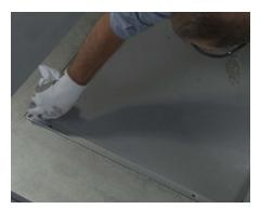
9 Use a rag to clean the excess grouting from the top of the frame leg. Allow
