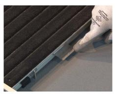
**11** Modules will have spacer clips attached to one side. Spacer clips should face toward adjacent modules.
