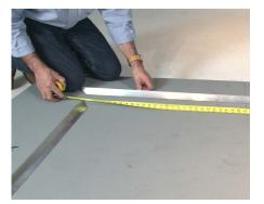
**1** Dry fit all frame pieces within the area and use a tape measure to ensure a proper fit. For odd-shaped layouts, match frame tags to the drawing on the pack list.
