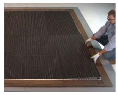
**12** Continue placing modules in the correct locations per the shop drawings.
