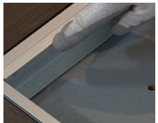
**3** The tread rails are at a1.5" on center increments. Filler bars may be required to achieve the exact overall dimension.
