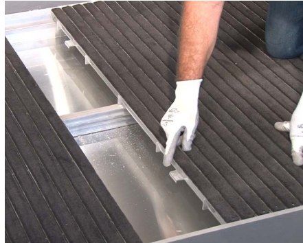
23 Make sure the attached locator clip is seated below the corresponding Pedigrid panel.
