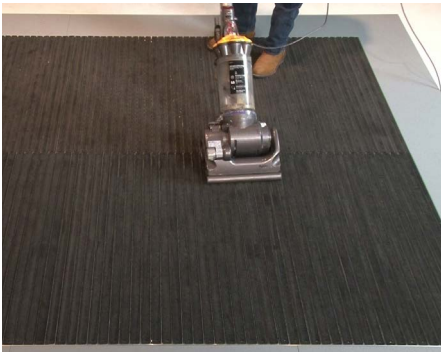
25 Clean the unit with a vacuum. If construction is to continue in the building, cover the unit with plywood sheathing.
