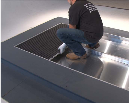
22 Place modules in the correct locations per the shop drawings.
