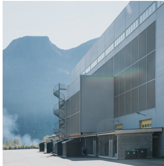
ARKON ENERGY DATA CENTRE GLOMFJORD, NORWAY PERFORMANCE LOUVRE
