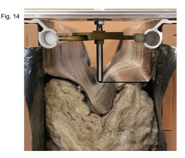
In Horizontal applications of TVB system, a layer of Vapor Barrier (7 ply.) material is installed over top the Thermal Vapor Barrier providing added protection to the elements.
