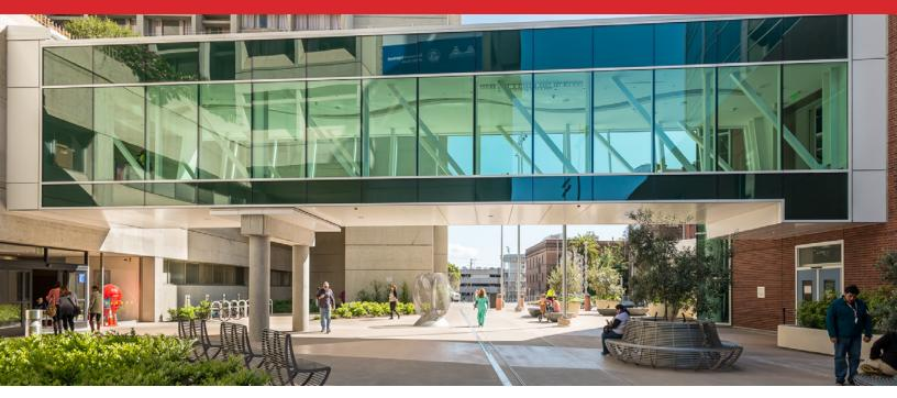
The multi-axial corridor cover (MACC) system seamlessly connects the new hospital tower to the existing structure, while the exterior moat covers visually unite the landscape and sidewalk.
