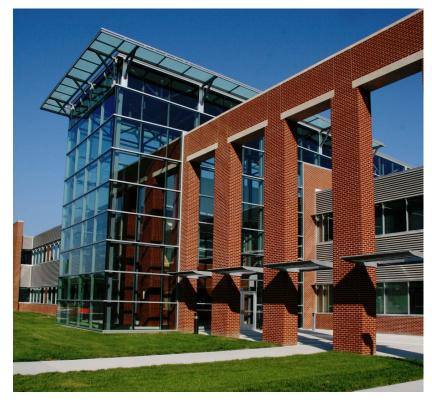
Lightshelves bring daylight deeper into the building, which has positive benefits on building occupants and reduces the overall building's energy costs, by reducing reliance on artificial lighting. Additionally increased insulation, external sunshades, windows that increase daylight and other innovations that increase the efficiency of mechanical systems are designed cut the building's energy demands by 20 percent.
