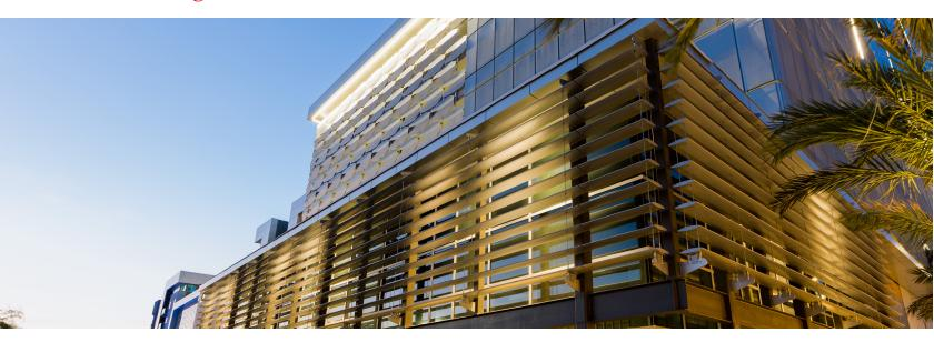
These sunshades come with an exciting "floating" effect. Supported with tensioned cables, the system can be quickly and efficently constructed on-site, thanks to the integrated aluminum collar.
