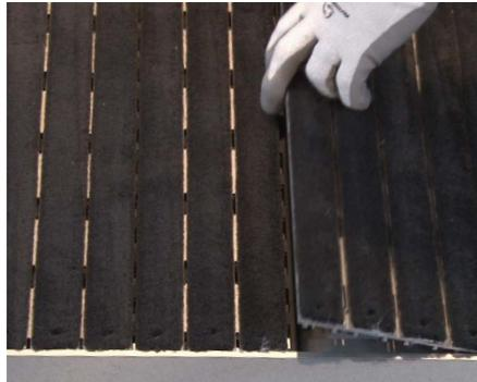
**5** Join modules together by placing the aluminum male foot into the adjacent module's female connector.
