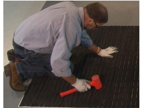
**6** Use a rubber mallet to join the foot into the connector.
