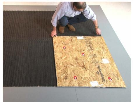
**12** If construction is to continue in the building, protect the unit with plywood sheathing.
