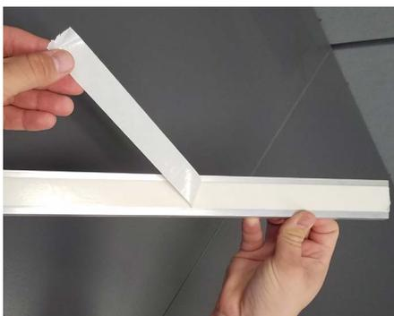
**3** Remove the covering on the tape and reinstall the frame in its correct position and location. Apply pressure on the frame to properly bind the tape to the flooring.
