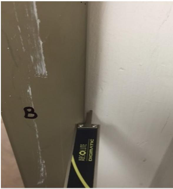
**Please note: Each door frame should be measured individually to verify that there are no dimensional differences from door frame to door frame.**
