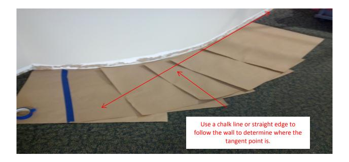
Tape all joints securely on both front and back sides to ensure that the templates hold up during the shipping process so we receive an accurate template. Use a scribe (compass) set at 1" and carefully follow the wall radius and transfer it to the paper. Cut with scissors along the line that you just made and verify that it fits the wall well. Repeat the scribe step if necessary until the template fits.
