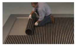
18. Care & Maintenance: to properly clean underneath the mat and avoid rail damage, roll back the mat edge to the 12th rail. Continue to roll back the mat holding that diameter.
