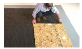
17. If construction is to continue in the building, protect the unit with plywood sheathing.
