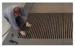
13. For beginners: we recommend using a straight edge to assist in cutting an accurate line. Once the end trim is adjusted, tuck the mat into the recess and push flat.
