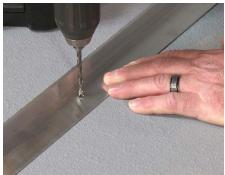
**3** Using the 5/16" masonry bit, drill into the concrete 24" on center. Fasten the frame with the supplied masonry anchors using a #2 Phillips-head screwdriver.
