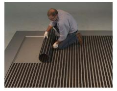
**16** Care & Maintenance: to properly clean underneath the grid and avoid rail damage, roll back the grid edge to the 12th rail. Continue to roll back the grid holding that diameter.
