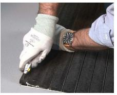
**12** For proper fit, the end trim can be cut in any of the grooves that are spaced 1/8" apart using a sharp utility knife. Score several times to cut
