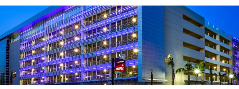
Airfoil Lux Sunshades function as a solar shading system during the day and light up at night to make an architectural statement. Energy efficient, low voltage LED lights inside a translucent polycarbonate nosing run along the front of the blade with millions of RGB color combinations. The 8" or 12" wide airfoil blades can be mounted in a vertical or horizontal orientation to create an architectural accent in both day and night.
